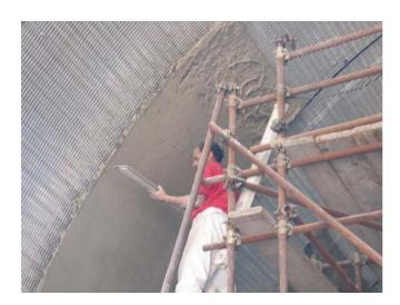
Despite high Summer temperatures, installation of the FireBarrier 135 lining was completed one month ahead of schedule and with material usage exactly in-line with the quantity estimated before installation.
