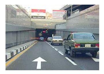
The Al-Azhar tunnel is a 2.5 km long twin tube concrete tunnel that runs under the city of Cairo close to the famous Al-Azhar Mosque. FireBarrier 135 was installed to the newly-built tunnel to protect the tunnel from collapse during a 1350 °C hydrocarbon fire of 2 hours duration (the RWS fire curve).
