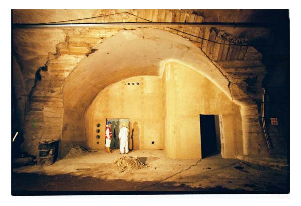
The FireBarrier 135 lining was installed in one single layer directly on the walls without the need for anchors or reinforcement mesh.
