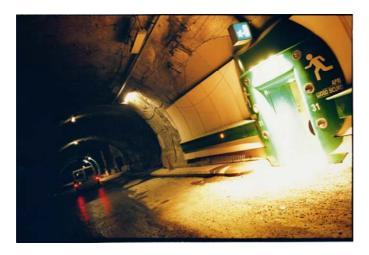
The refuges are built into the rock adjacent to the tunnel and are built from blockwork brick onto which FireBarrier 135 was sprayed to provide fire protection. Two different levels of fire protection were required for the refuges:
