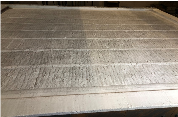
Figure 1: Newly installed Superwool Prime Pyro-Fold™ Modules
