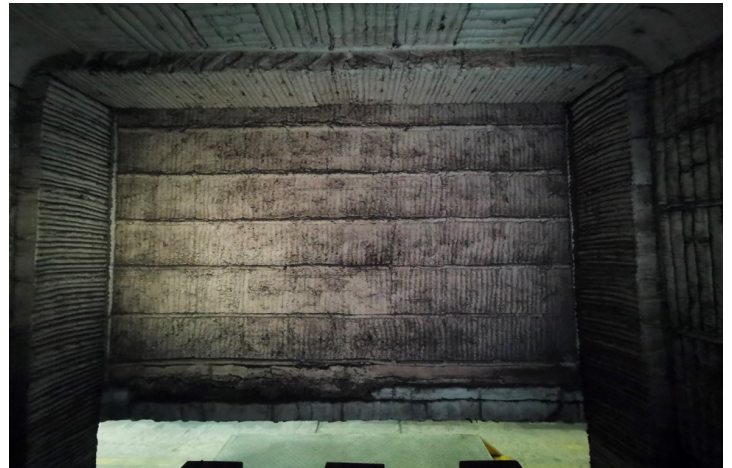
Figure 2: Superwool Prime Pyro-Fold Modules, after 6 months use
