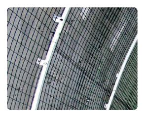
FireBarrier 135 is normally installed by spraying over a mesh, which is fixed to the concrete lining using "pig tail" anchors.
