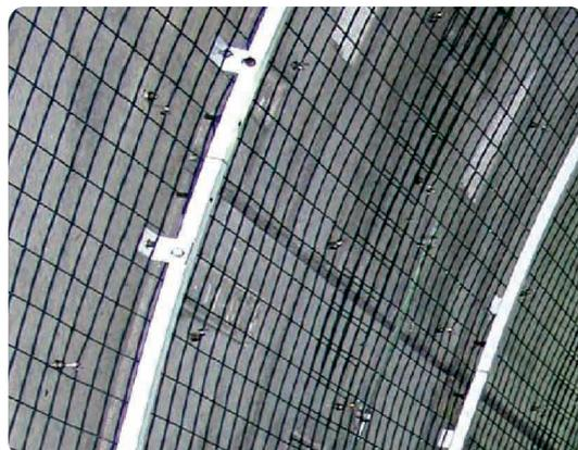
FireBarrier 135 is normally installed by spraying over a mesh, which is fixed to the concrete lining using "pig tail" anchors.
