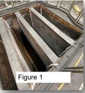
The pit walls in the ABF (Figure 1) are manufactured from dense refractories and insulating bricks. Unfired anode blocks comprised of coke and pitch are lowered into the pits and completely covered with powdered coke.
