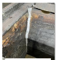
Superwool Prime installed into expansion joints
