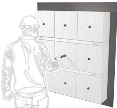
After installation of the module REMOVE TUBE. Pyro-Bloc M Modules - red plastic access tube
