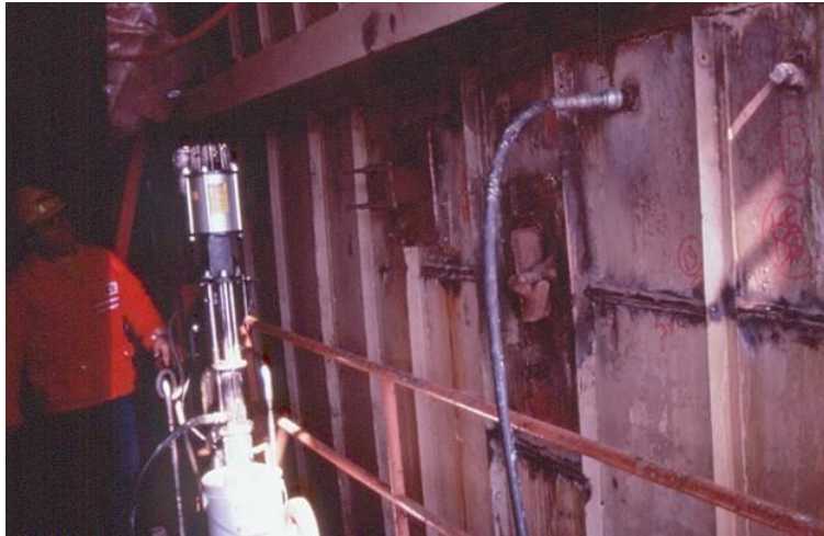
Figure 2 Installing Pumpable into the hot spot while furnace remains online
